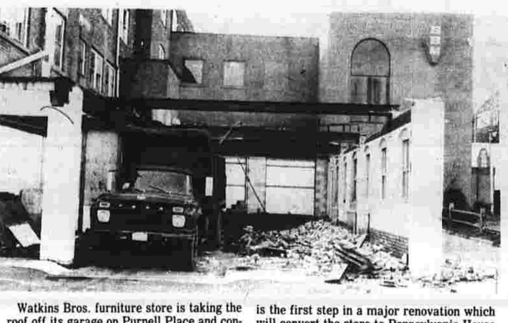
Watkins Bros. furniture store is taking the roof off its garage on Purnell Place and converting it to a walk-in loading area for large trucks, including tractor-trailers. For more trucks, see page 14.
